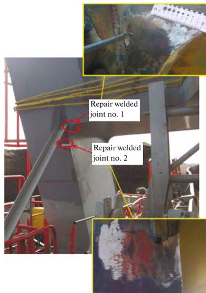
**Fig. 15.** Examined repair welded joint at the structure of the left column of the P frame, internally designated with nos. 1 and 2.
