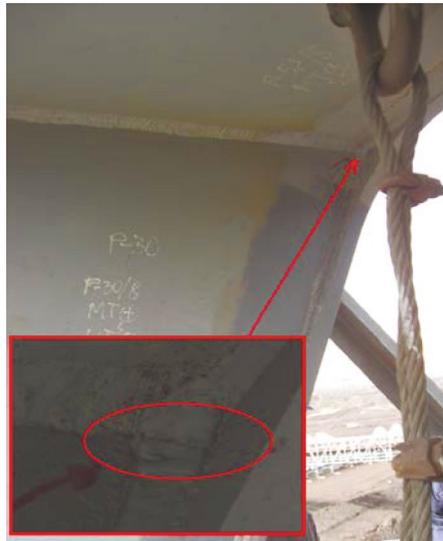
**Fig. 3.** Cracks on the surface of column fillet welded joints—right side (crack lengths up to  $L = 20$  mm).
