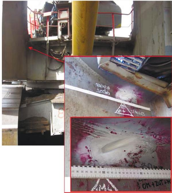
**Fig. 11.** Grinded section at the right side of the rotating platform.
