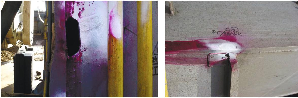
Fig. 7. Damages at parent material and welded joints of the P frame—left side.
