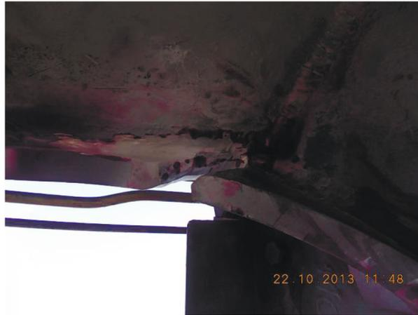
**Fig. 9.** Grinded fillet weld at the right column of the P frame (detail B at Fig. 10).
